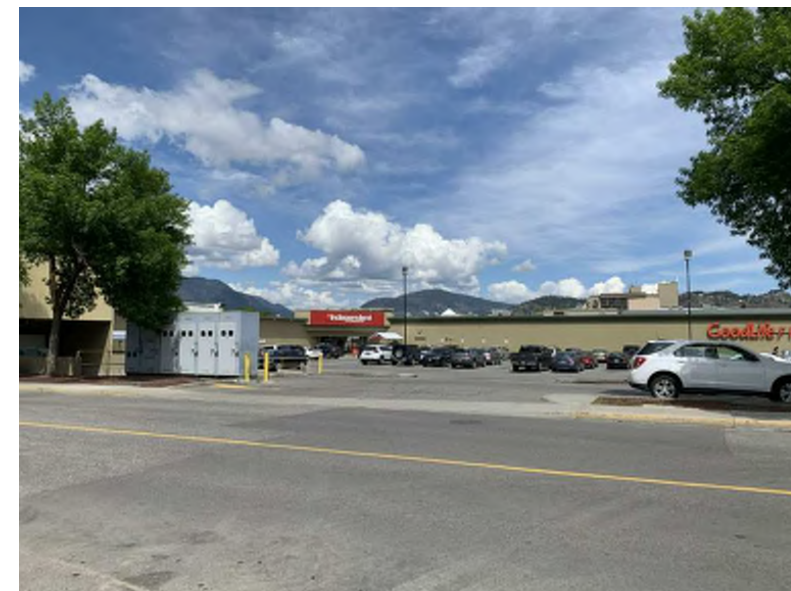
6. LOOKING NORTHWEST TOWARDS PROPOSED SERVICE ROAD ENTRANCE
